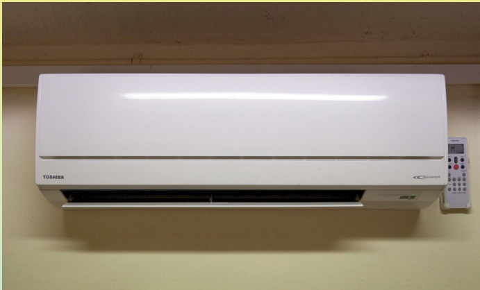
R410A split air-conditioning unit converted to RS-53 (R470A) & operating satisfactorily without any problems
